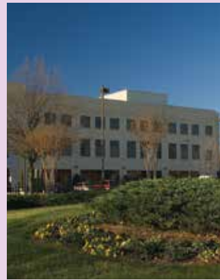
Richmond Community Hospital 1500 N. 28th Street Richmond, VA 23223 804-225-1700
